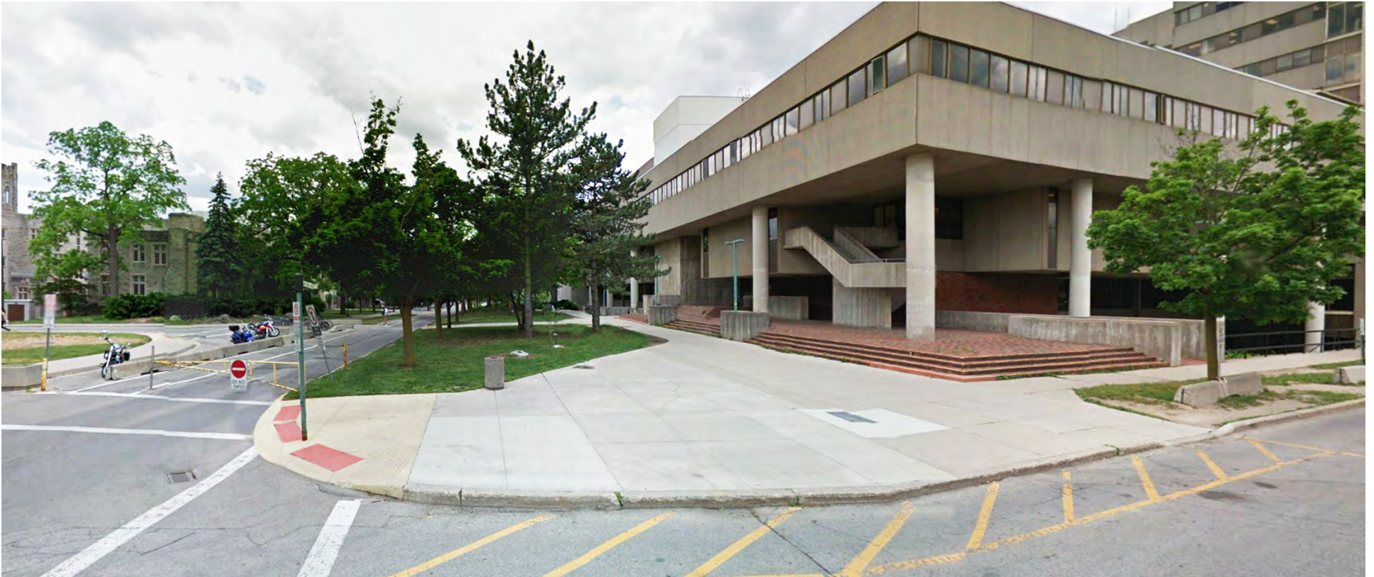
Existing conditions: Social Science Plaza
