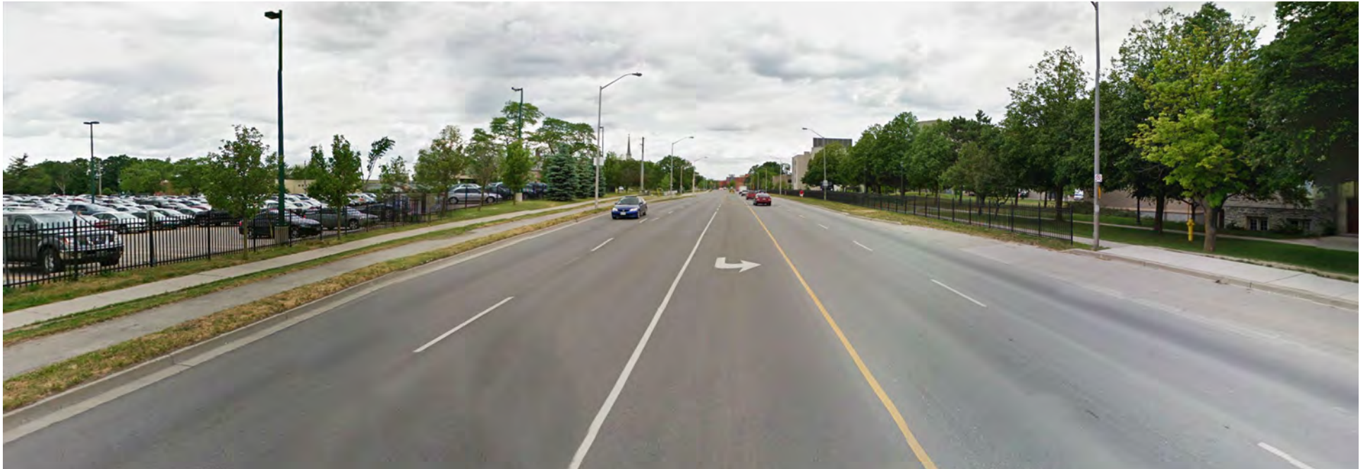
Existing conditions : Western Road at Springett Parking Lot
