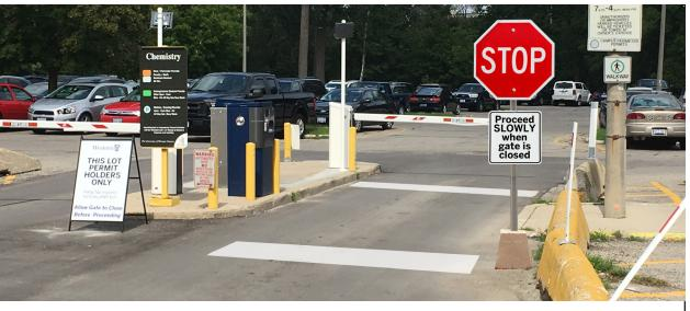
exit lane. You will see the light array on the hang tag reader on the white pole change colour as your vehicle triggers the detectors below the entrance.
