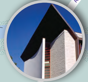
10 John Labatt Visual Arts Building 1993 This building is home to Western's Fine Arts program. Many varied art displays can be seen within and without.
