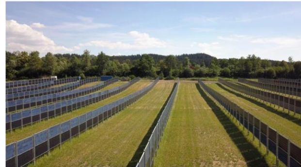
Agrivoltaics is a relatively new field that involves combining solar photovoltaic panels in agricultural operations. (Tobi Kettner/Wikimedia Commons)
